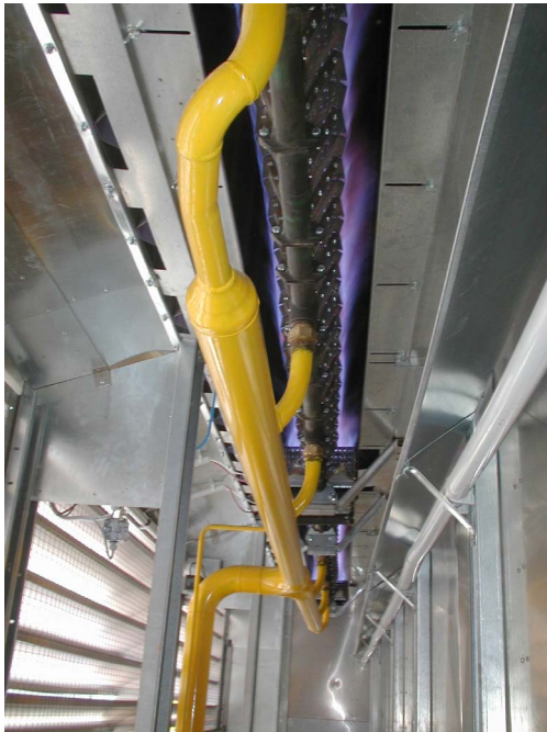
Direct air heating with AHP AIRFLO® burners in continuous flow dryers for grain
